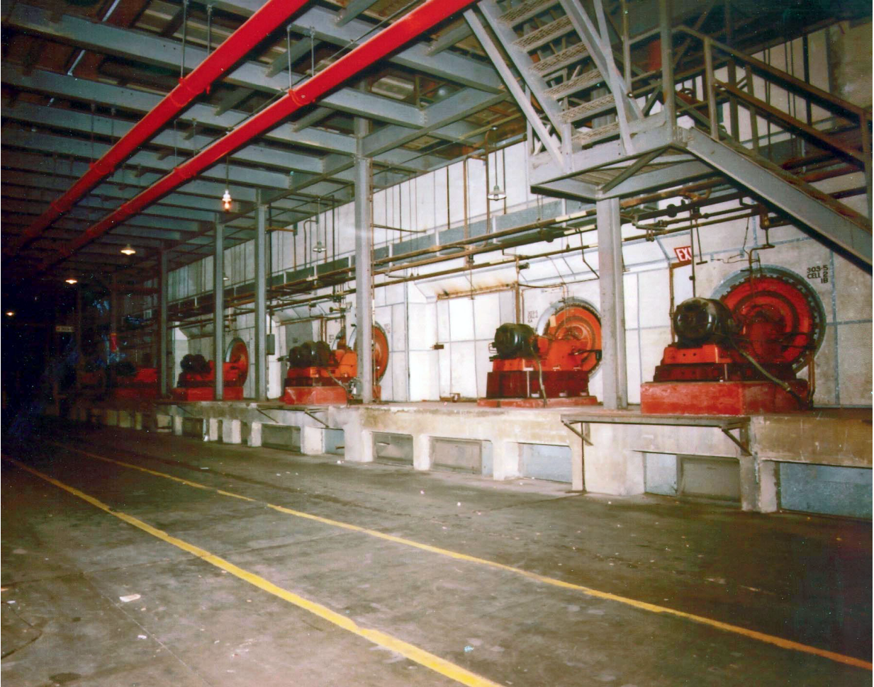
A view of the actual motors and pumps that moved the uranium gas through the series of cells – this view conveys the size of the facility and the number of gaseous diffusion stages in each alley
